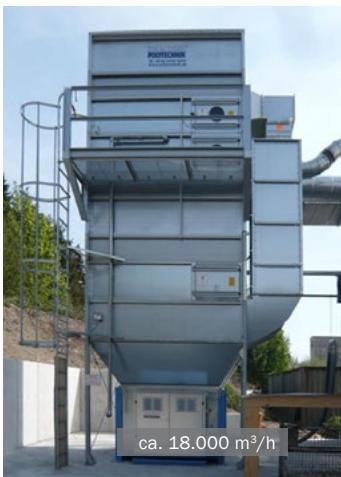
MultiStar Pressenfilter • Innenausbau
