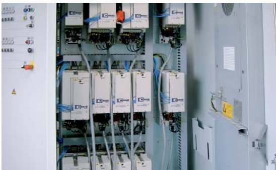
Free-standing switch cabinet with refrigeration unit and separate frequency converter per motor
