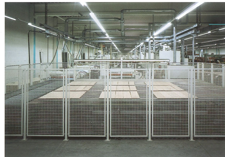
View of the complete finishing plant with grid transfer
