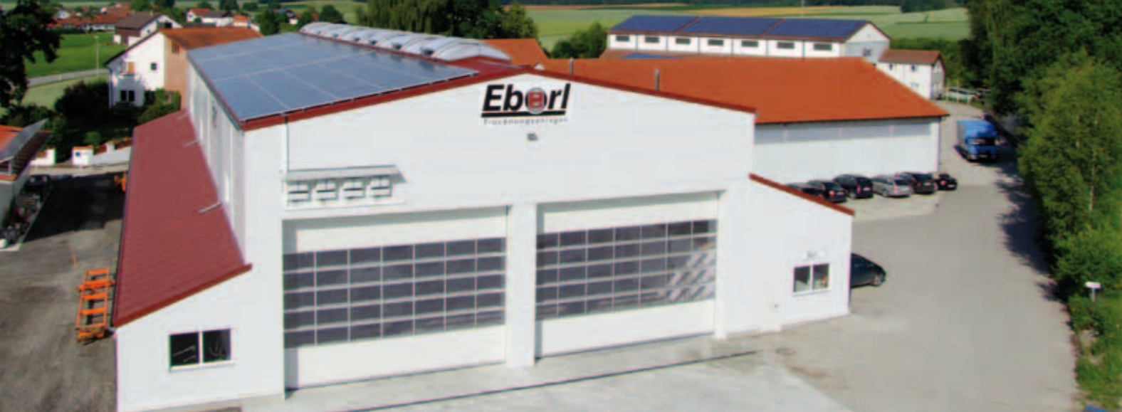
EBERL premises in Bodenkirchen, Bavaria / Southern Germany.
