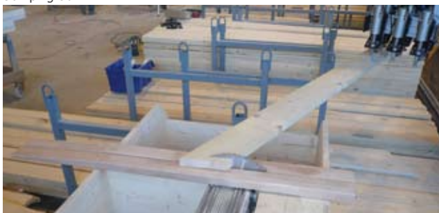
trimming of too long boards
