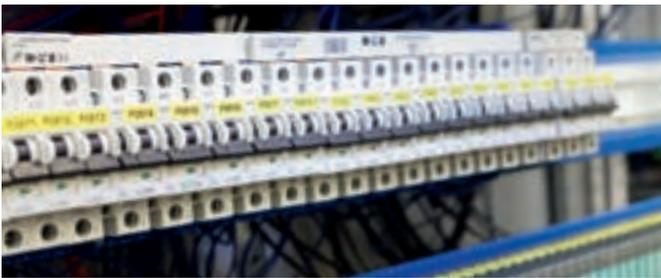
The designation of equipment is structured logically and arranged according to function. Each component in a WEINIG switch cabinet has a fixed designation. If a fault occurs, the WEINIG service team only needs the alpha-numeric name of the unit from the customer. An invaluable advantage which ensures that your machine will be quickly back in production.
