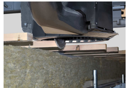
Formatting the roof battens
