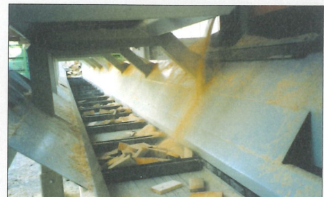
Waste evacuation systems
