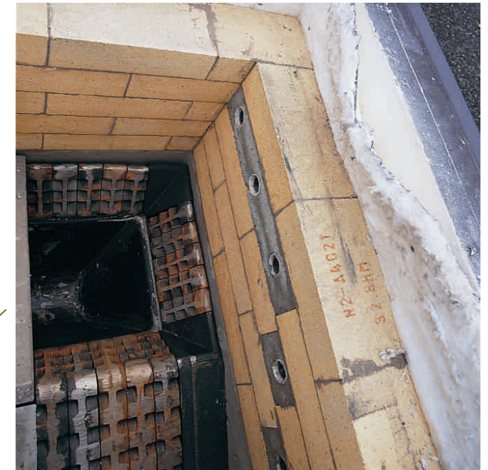
Combustion chamber design - unique multi-sectional insulation and high quality brick refractory lining
