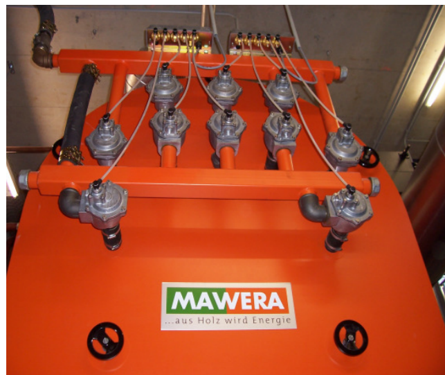
Soot blower for cleaning heat exchanger (optional)
