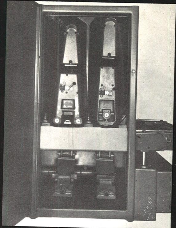
1 - Control side showing belt tracking and oscillation equipment and roll adjustment system to be used for slightly bell-shaped belts.
