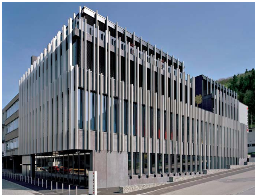
Built corporate identity: Vertical aluminium pilaster strips subdivide the front of our principal office in Littau in the near of Luzern, and establish a good reference to our products and market partners.
