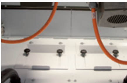
Supportive room extraction
