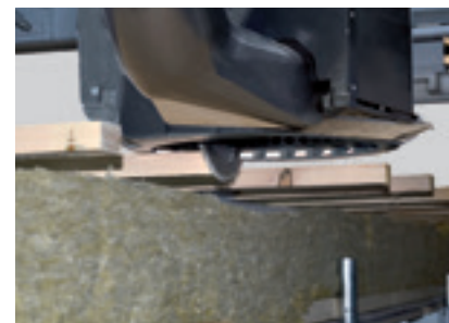
Formatting the roof battens
