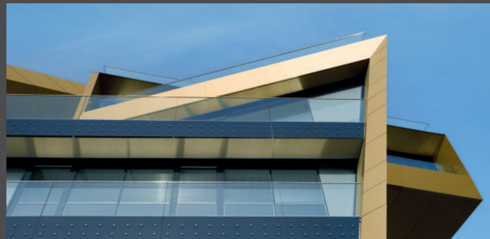
The ALUCOBOND® aluminium composite façade in gold metallic evokes associations with coins or with the bank's corporate identity.
