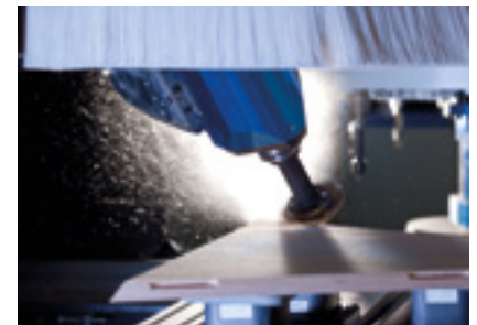
Trimming of inclined grooves for panel connection
