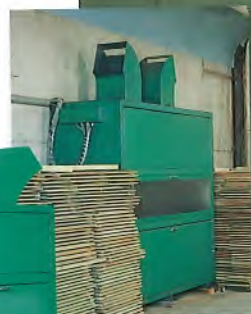
▲乾燥窯內部安裝情形 Dry Kiln Inside Installations
