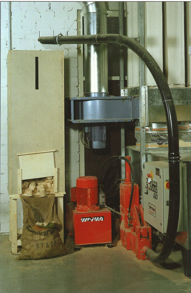
Retrofit under a bag filter system
