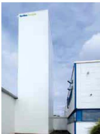
To increase the existing facility capacity, the Shuttle XP devices can be installed outside the building and skilfully walled in with a pass-through access.
