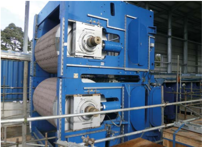
Installation: Inverness, Scotland
