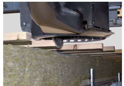
Formatting the roof battens
