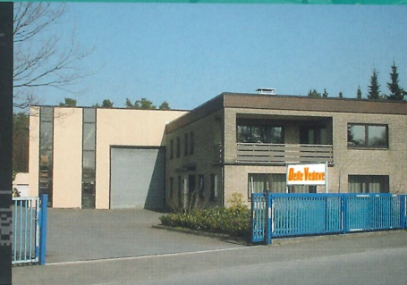
New plant in Schloss Holte
